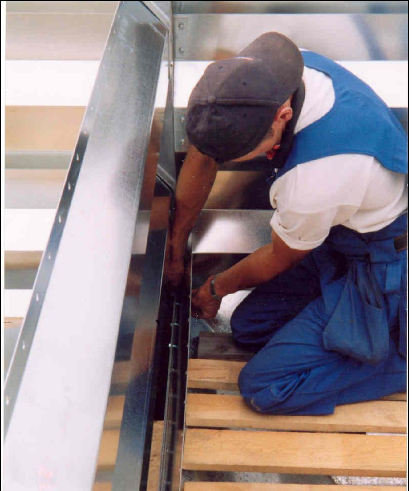
Installation of the silo cone spacer plates.
