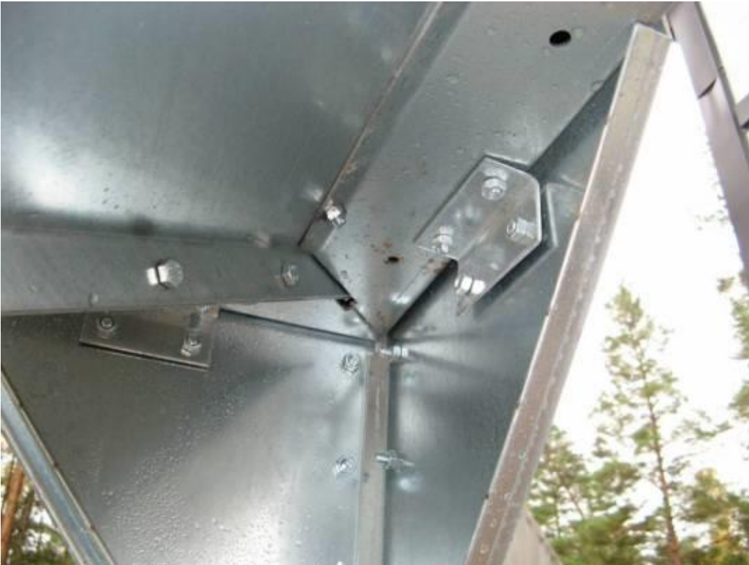
A photo showing the fastening of the central leg to the cone. The arrows point to the topmost row of perforation without bolts inserted.
